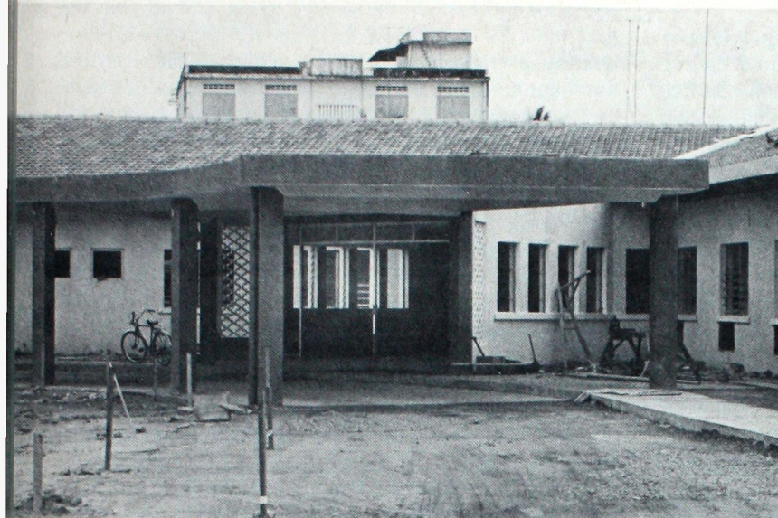
The Christian hospital shortly before completion
